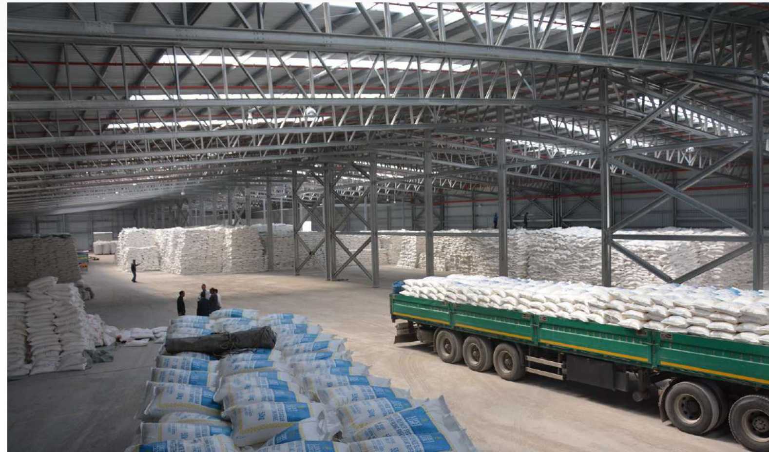
Pelit Antrepo Port Warehouse - Kocaeli, Turkey
